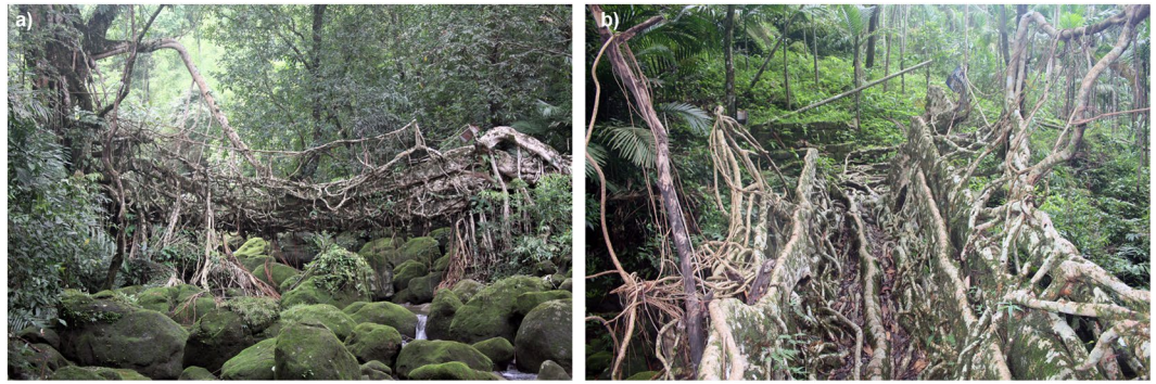
Figure 1. (a) Ummonoi Bridge, with a span of 7 meters, is a typical example of a mature living root bridge. Other bridges have spans up to 53 meters. (b) is taken from the centre of the bridge, looking towards the right-hand end of (a). (bridge #57 in Table S1 in Supplementary Information).
