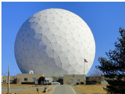
(b) Metal space frame radome
