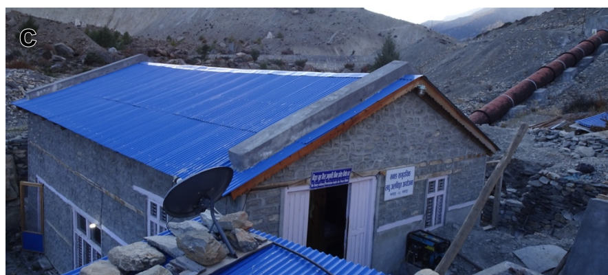
Figure 2-15: MHP power house with penstock (a & c) and vertical Francis turbine with generator (b) [Own Illustrations]
