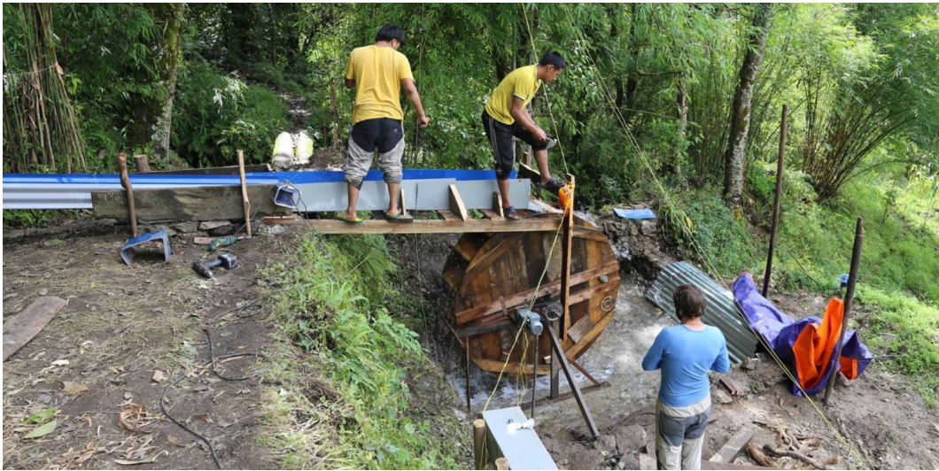
Figure 5-3: Prototype of a low-tech water wheel set up in the Solo Khumbu area in Nepal [Stephan Baur]
