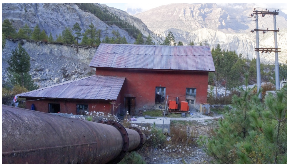
Figure 2-13: Sabje Hydropower Plant with its penstock [Own Illustration]
