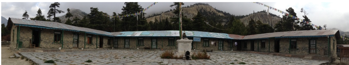
Figure 4-23: School 1 – Lophelling Boarding School: Classrooms [Own Illustration]
