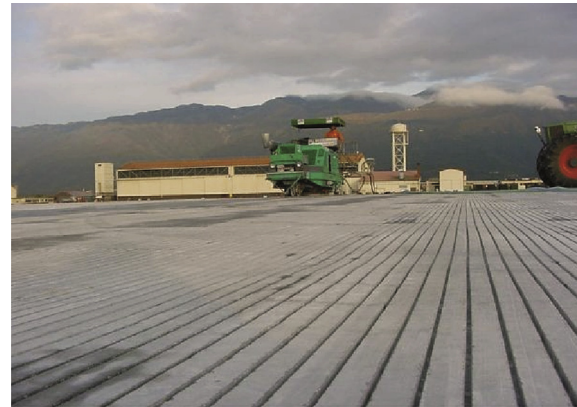
Fig. 3 – Diamond grooved texture (source: Otto Alte-Teigeler GmbH).
