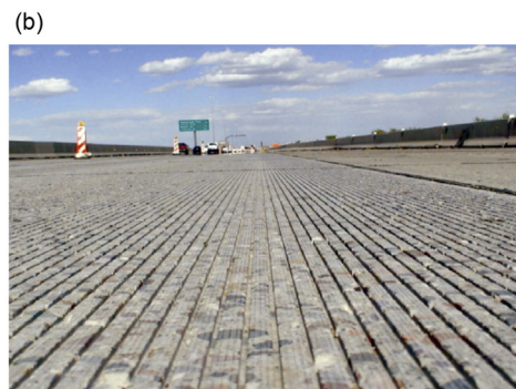
Fig. 5 – Cutting head and produced NGCS. (a) Cutting head for NGCS (for a single pass operation). (b) NGCS texture (IGGA, 2014).
