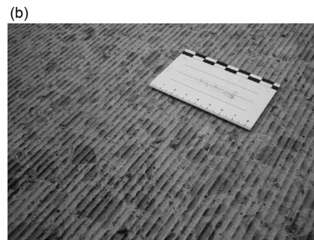
Fig. 2 – Cutting head and typical surface texture. (a) Grinding head. (b) Typical diamond ground texture.
