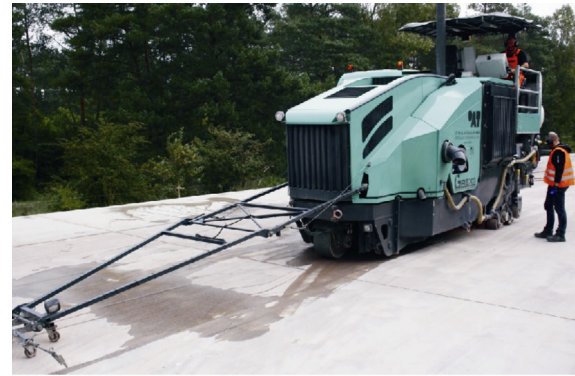
Fig. 6 – Diamond grinding in Germany.
