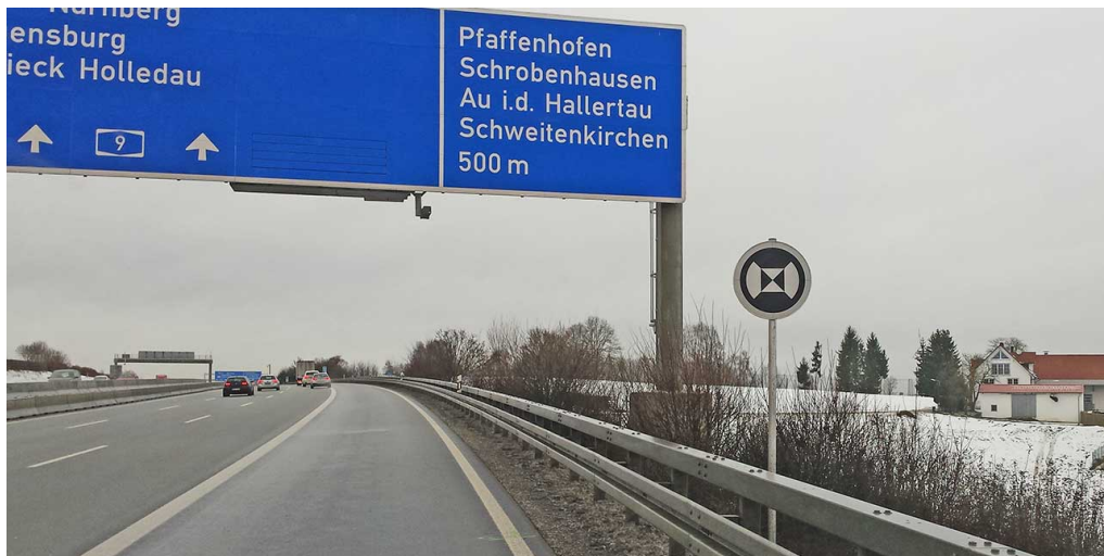
Figure 16 These signs are put up along a section of the autobahn A9 in order to support accurate positioning of vehicles (Picture taken from [43])
