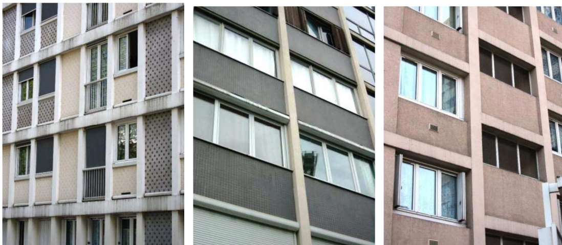
Figure 19. Type F4 facades.
