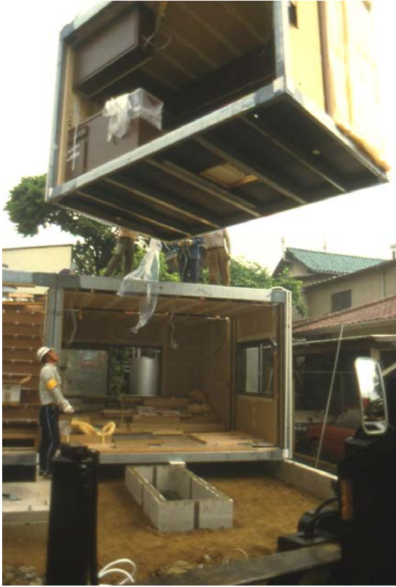
Figure 11: On-Site assembly of 80% prefabricated House
