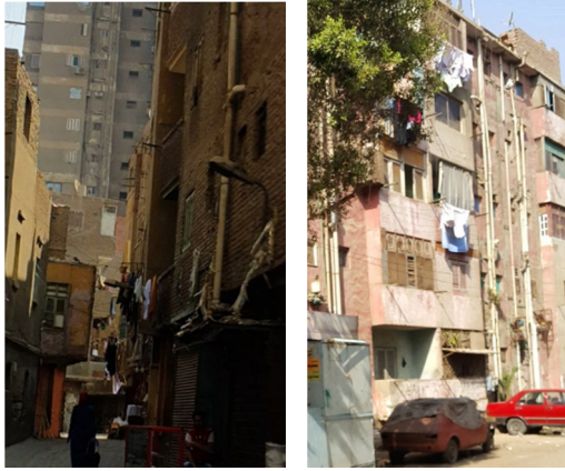
Figure 6: Low sanitation conditions in Farahat street (left) and 6 th October street (right) (Image: M. Sc. Maged Helal).
