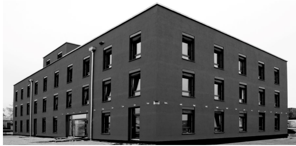
Figure 19: Ferdinand Tausendpfund GmbH & Co. KG office building, in Regensburg, Germany built in 2017. It has three storeys and is 27m long, 14.7m wide, and 9.8m tall. The gross volume is approx. 3950 \text{ m}^3 , with a gross area of 1290.5 \text{ m}^2 and a window-to-wall ratio of 25%
