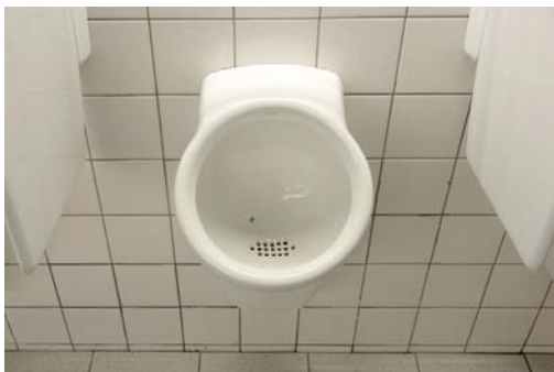
Figure 19 A fly on men’s room urinals, illustrating a non-digital trigger to avoid spillage. Retrieved June 21, 2017 from https://worksthatwork.com/1/urinal-fly
