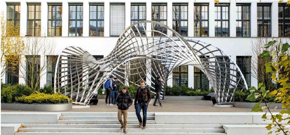
Figure 16: The Asymptotic Gridshell was completed in October 2017. The structure is 5 m high and spans 9×12 m. It is built entirely from 1.5 mm thick and 100 mm wide steel lamellas.
