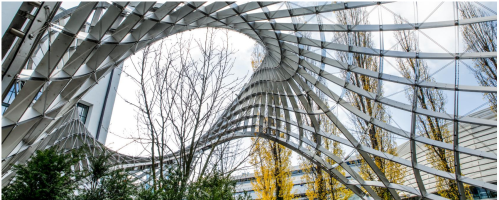
Figure 1: Inside the 'Asymptotic Gridshell'. It was designed for a green courtyard, encompassing a central tree. The strained gridshell was assembled with orthogonal nodes, from straight and flat lamellas, and erected elastically.
