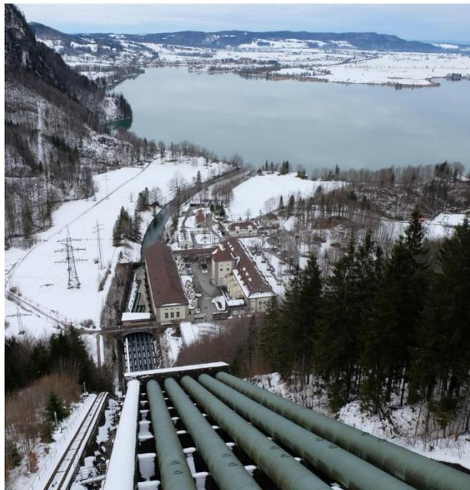
Figure 26 Penstock and machine house of the Walchensee power plant and the lower reservoir Kochelsee in southern Germany constructed in 1924 with an installed peak power of 124 MW
