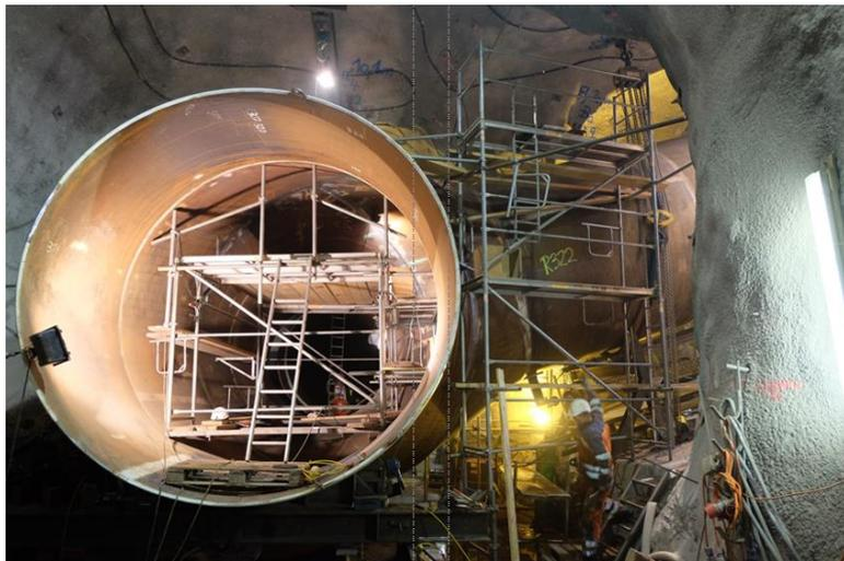
Figure 27 Penstock under construction for the Obervermuntwerk II in alpine Austria with a planned peak power of 360 MW and a flow through of 160 m<sup>3</sup>/s
