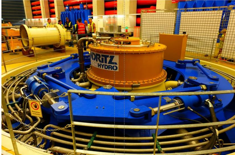
Figure 28 Six nozzles Pelton machine with a peak power of 150 MW, a flow through of 25.3 m<sup>3</sup> and a water velocity at the injectors of 450 km/h as a part of the Kops II power plant constructed in 2008
