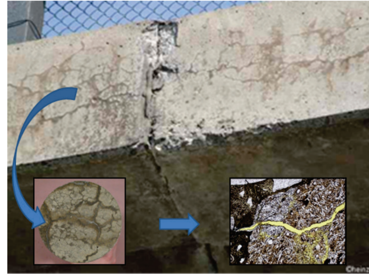
Figure 1: ASR damage due to deicing salt and procedure of diagnosis
