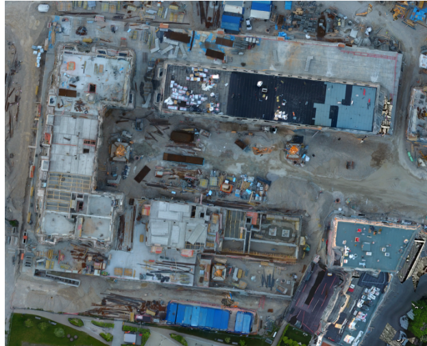
Figure 7: Top view of the construction site
