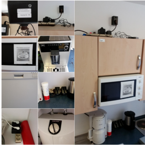
Figure 5.1.1: Appliances connected to open energy monitor in kitchen
