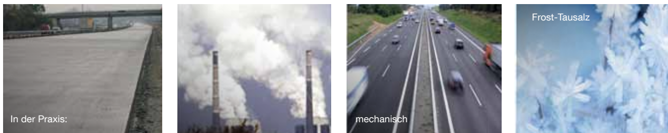
Figure 2: Types of exposure on concrete traffic surfaces
