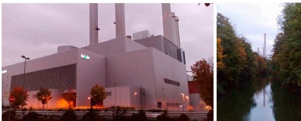
(a) External view of the building (b) View of the chimneys from far away
