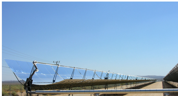
Figure 1.1: A parabolic trough solar collector [61].
