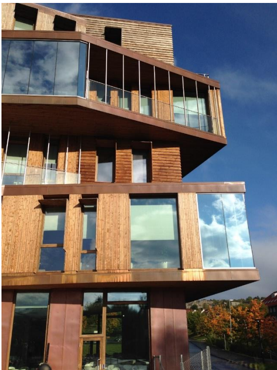
Figure 1 Exemplary urban tall timber building with a complex building envelope showing many critical spots in facade connections.
