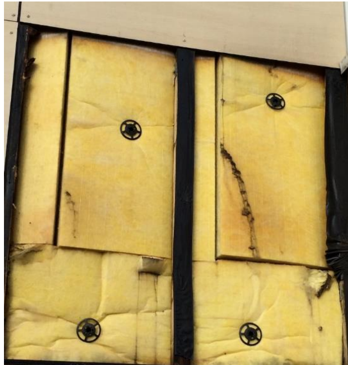
Figure 21 Wet mineral wool insulation – FCBA expertise.
