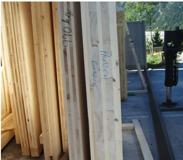
Figure 12: The elements on the parking place
