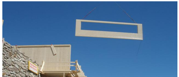
Figure 14: The window coming by helicopter and the view from inside
