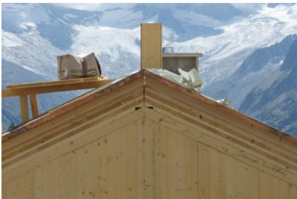
Figure 6: Wall and roof
