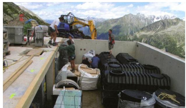
Figure 16: Installing the equipment in the basement
