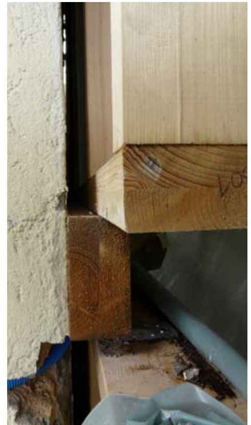
173. Beam carrying the load to the first floor ceiling.
