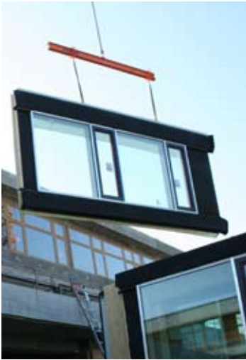
8. Prefabricated façade element assembly at Realschule Buchloe.
