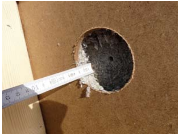
111. Hole for control of filling
