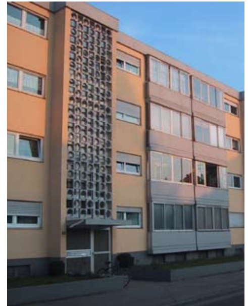
45. Curtain wall at stair case, loggia with additional glazing for noise protection, D-Augsburg
