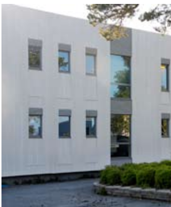
6. Risør College, Norway Prefabricated façade elements with close boarding, assembled in 2009.
