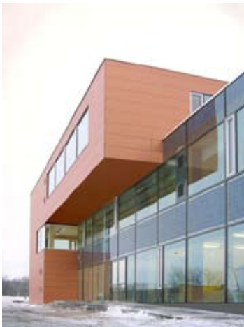
5. Schwanenstadt, Austria School before and after modernisation; PAUAT Architekten, 2004
