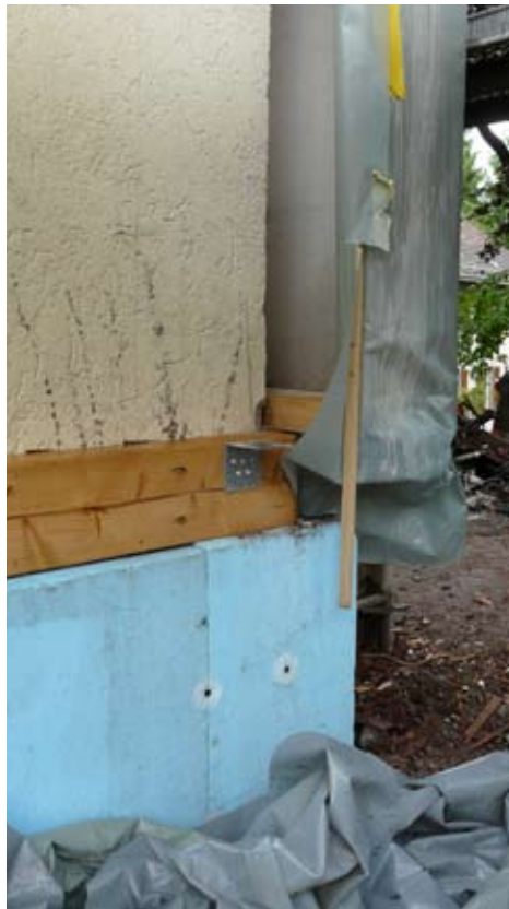
172. Basebeam with styrofoam insulation
