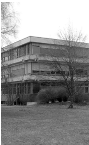
186. Existing school building
