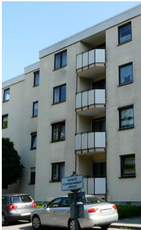
55. Partly cantilevered slab
