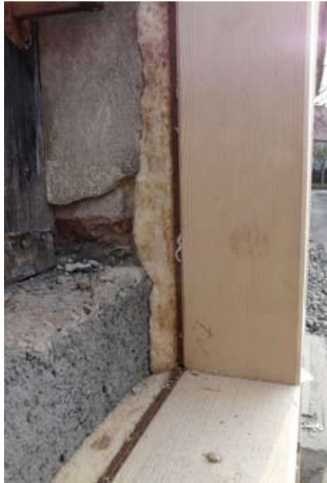
107. Window sill and reveal with sealing.
