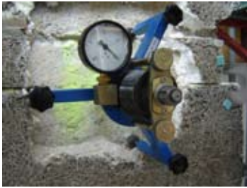
134. Pull test at an existing concrete wall.
