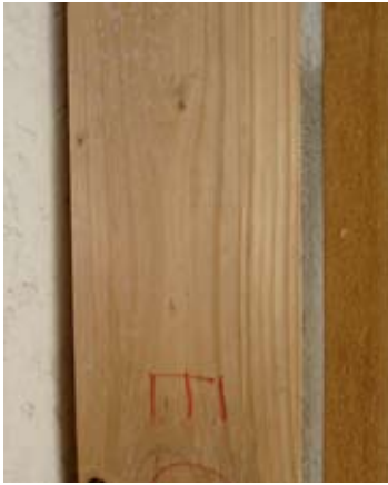
170. Layering of element in front of existing wall (left side).
