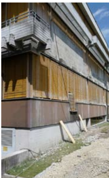
190. Demolition of balconies and old façade
