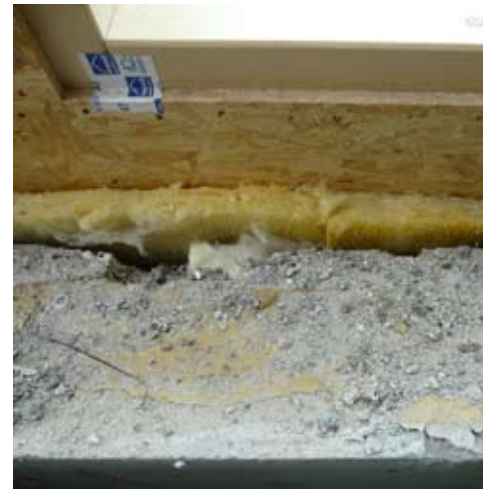
102. Element joint at sill
