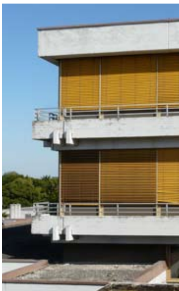
189. Before modernisation - concrete balconies
