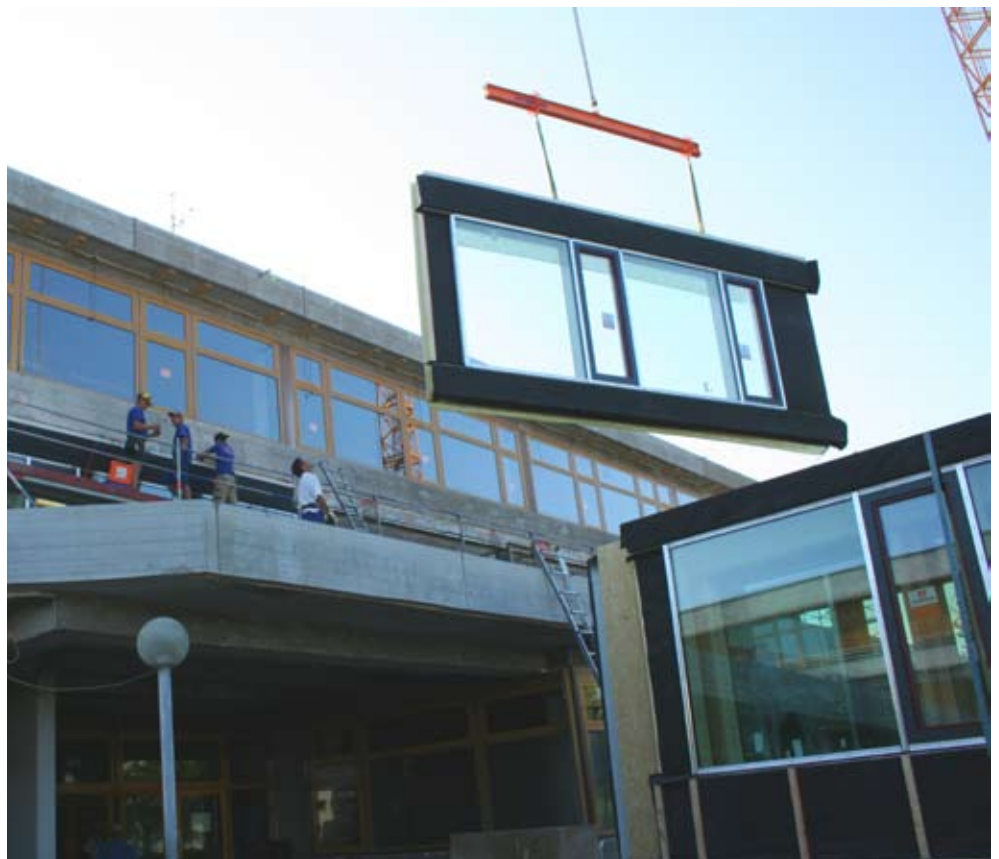
193. Mounting of TES elements
