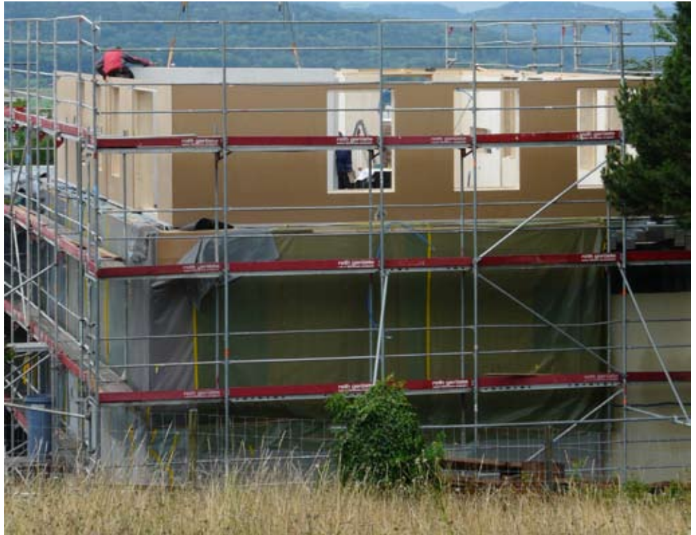
171. Roof extension of existing apartment block.
