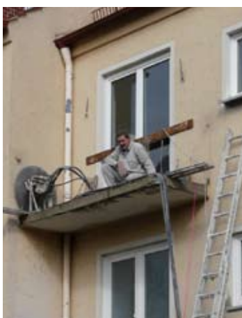
57. Cutting off balcony slab
