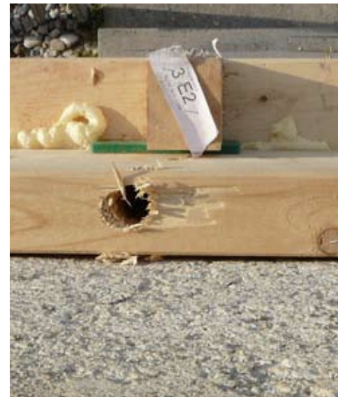
113. Drilled hole for filling hose.
