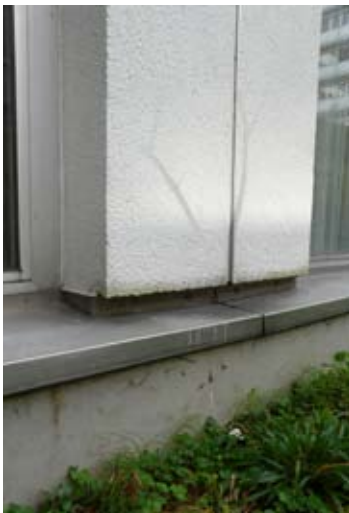
34. Joint in concrete skeleton structure
