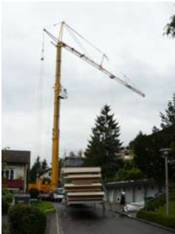
167. Transport of lying elements on bridge plate.
