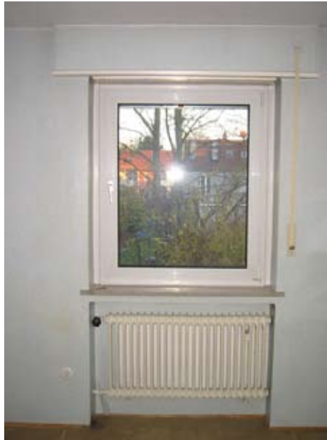
42. Interior rolling shutter box and radiator niche, brick masonry 30 cm, D-Augsburg
