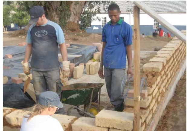
Figure 8: students working on clay brick wall
