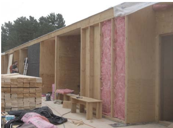
Figure 10: exterior timber framed wall with insulation
