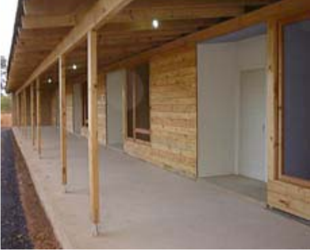
Figure 4: view of covered outdoor space in front of the play rooms
