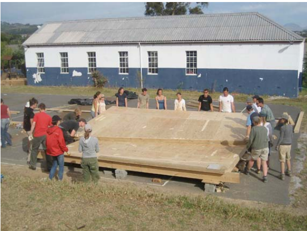
Figure 5: prefabrication and transport of timber wall
