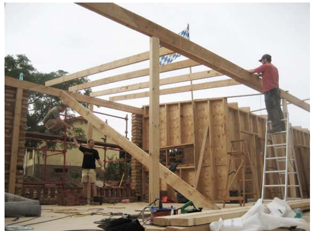
Figure 6: raising of the rafters of the roof construction
