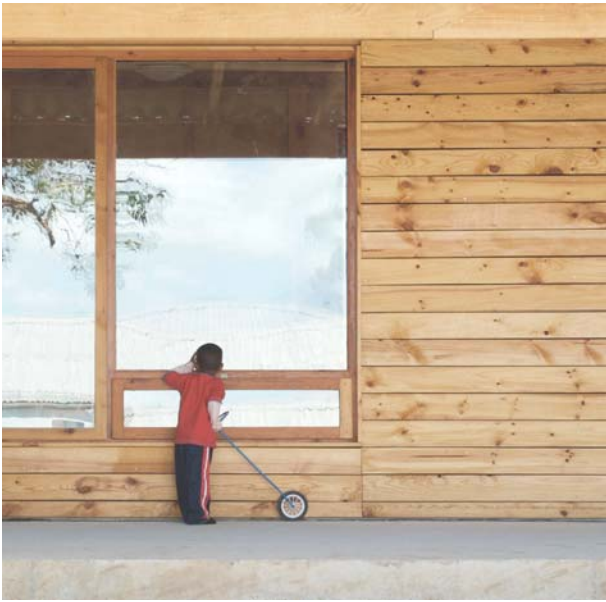
Figure 13: show-case window with low set casement in the South facade (photograph: M.Hall, Cape Town)
