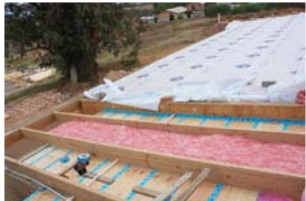
Figure 11: roof during construction with insulation and permeable under-tile membrane
