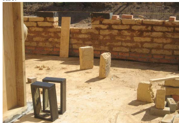
Figure 9: black wooden boxes later used for fixing window frames
