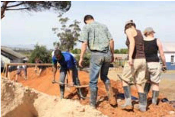
Figure 7: mixing the clay mortar
