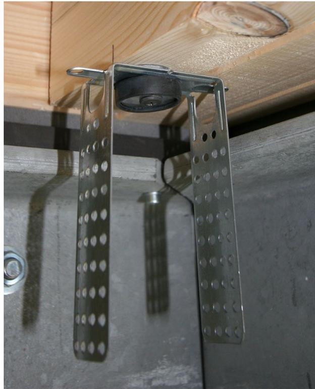
**Figure 4.15:** Sound insulation hanger
