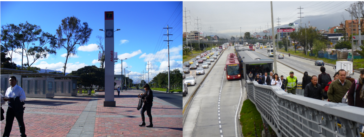
Figure 4.4 Alcalá TM station. Source: (Transmilenio, 2015a)
