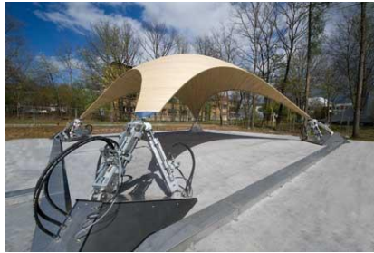
Figure 1.2: The adaptive "Smart Shell" structure in Stuttgart (source of picture: [127])
