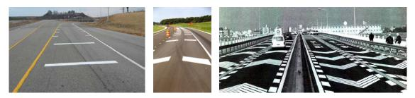
**Figure 3.15:** Pavement markings for speed manipulation. The left and middle markings were developed by Katz in [Kat07] and are installed in the USA, the chevrons in the right image served as basis for the work of Drakopoulos in [Dra03] and are installed in Japan.
