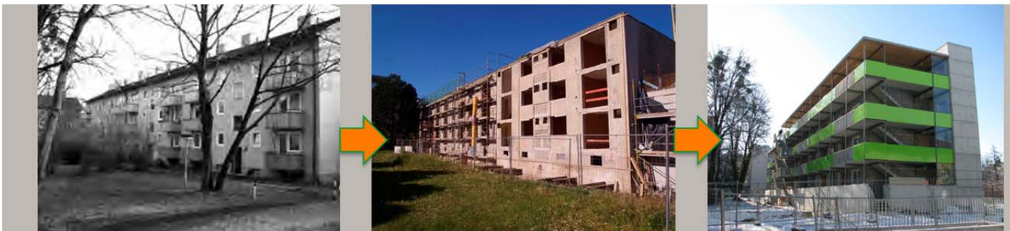
Figure 2-14 Process of change from original building, refurbishment site process, to end result GWG Munich (photos GWG archive, le Roux, Ott)
