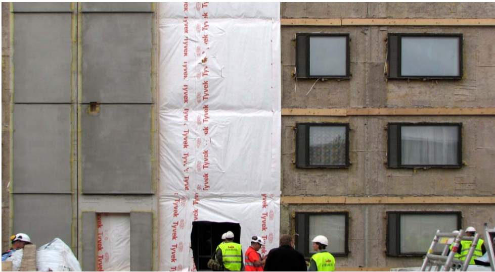
Figure 1-7 TES energy facade in Riihimäki, Finland. (photo: le Roux, 2011)
