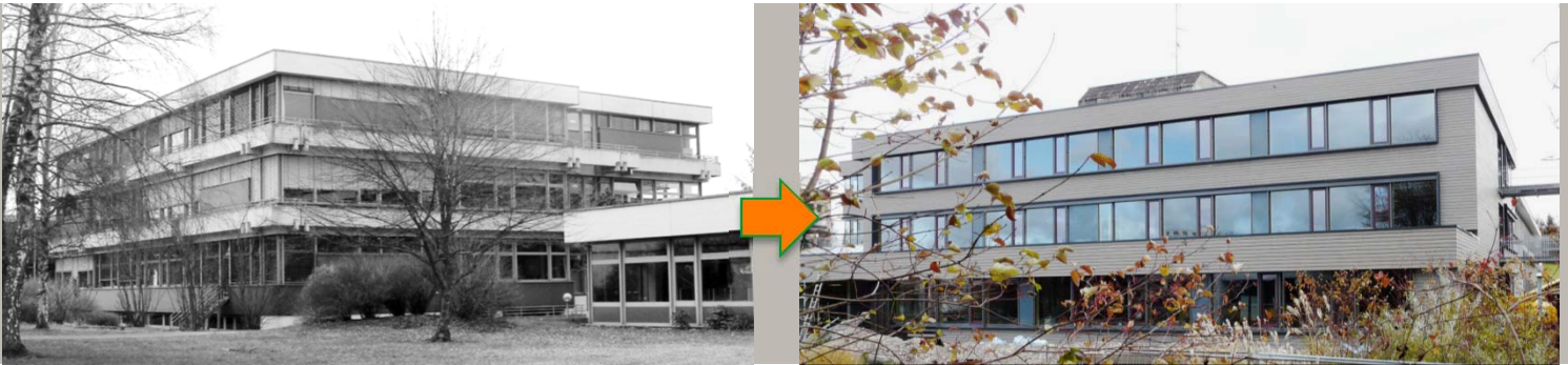
Figure 2-20 Process of change at Realschule Buchloe from original building to end result with TES facade (photos Ott)
