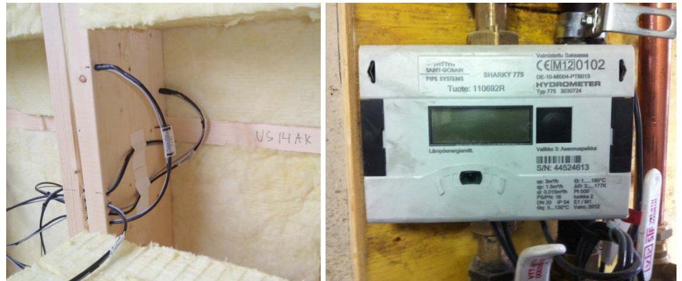
Figure 1-15 Monitoring building physics and heating energy after TES retrofit for E2ReBuild demonstration project in Oulu, Finland. (photos: Karhumaa (Fidelix), and le Roux, 2012)
