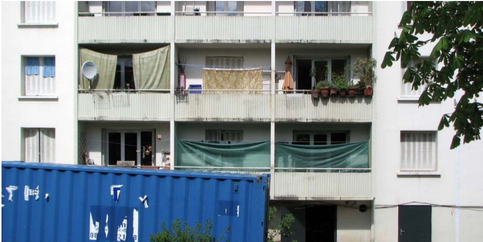
Figure 1-13 Housing undergoing energy retrofit in Voiron, France. (photo: le Roux, 2012)
