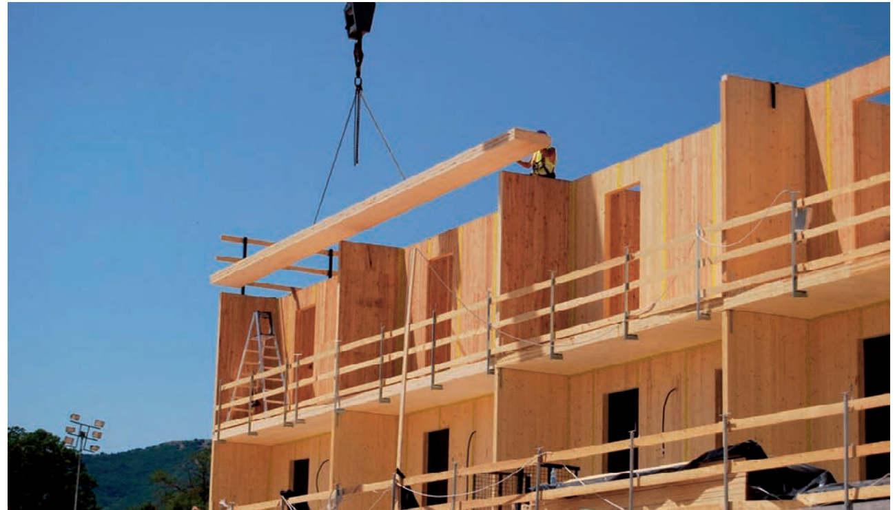
F.6.6 Construction site, L'Aquila building, Italy
