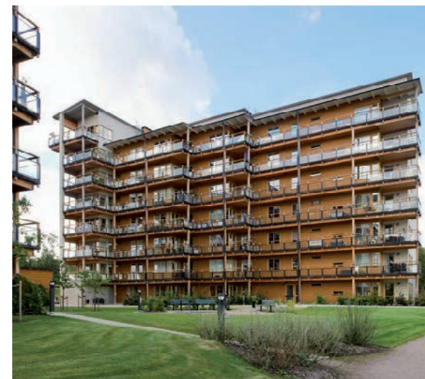
F.3.6 An award-winning 8-storey CLT-frame building in Växjö, Sweden
