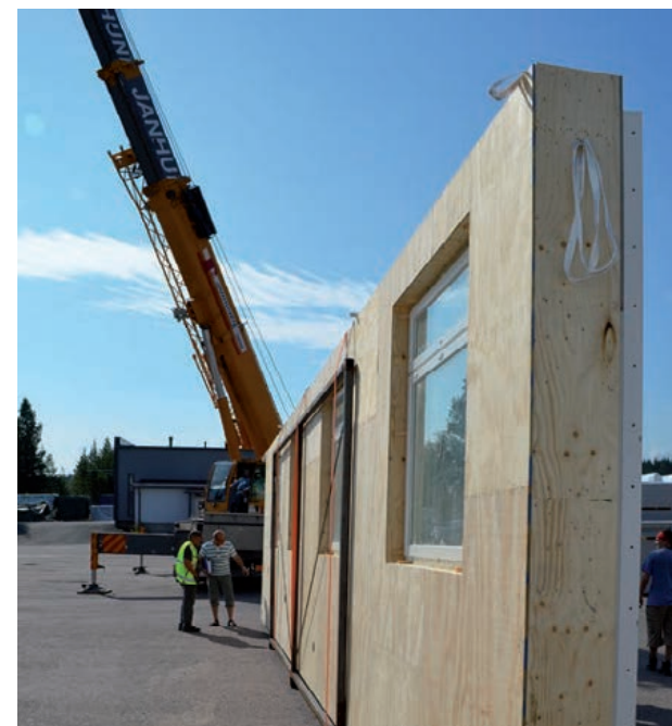
F.4.5-10 Installation of a TES-element, Finland
