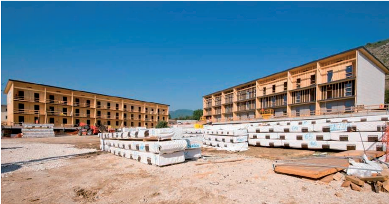
F.6.3-13 Progetto C.A.S.E, construction site, L'Aquila, Italy
