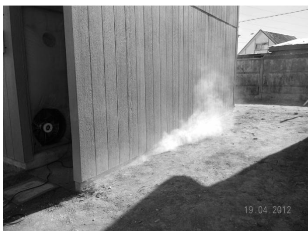
Figure 2: Smoke test performed to a timber house
