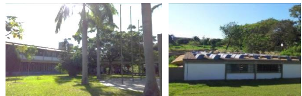
Figure 3: Vegetation (a) and roof openings (b)
