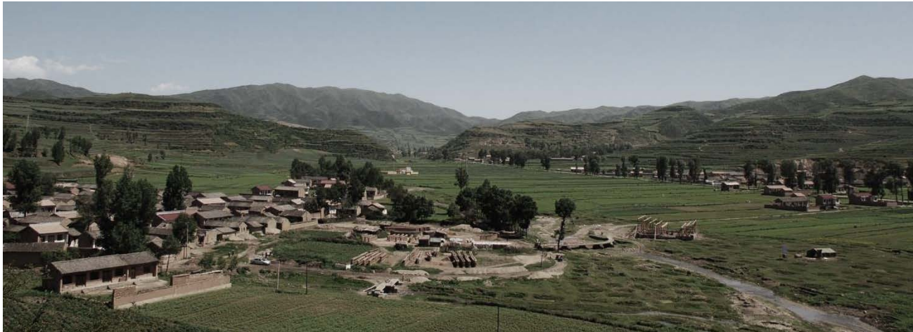
Figure 3: Overview of the village and building site.
