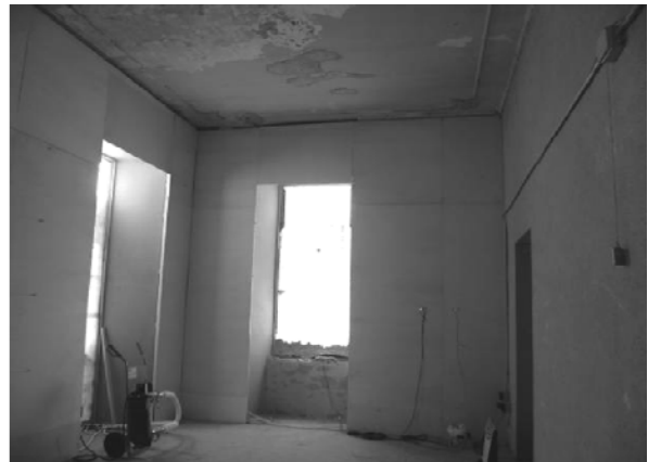
Figure 2: Experimental room in the building called "ex Casa Gramsci"
