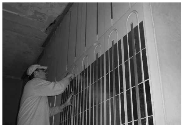
Figure 3: Anchorage of the insulating/radiant panels in the experimental room
