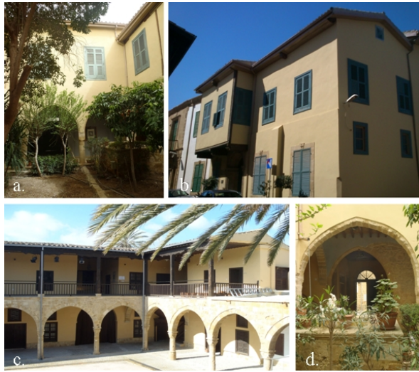
Figure 3: General views of exterior and semi-open spaces of the selected study buildings. (a, b and d: Student Hostel c: Cultural Centre).
