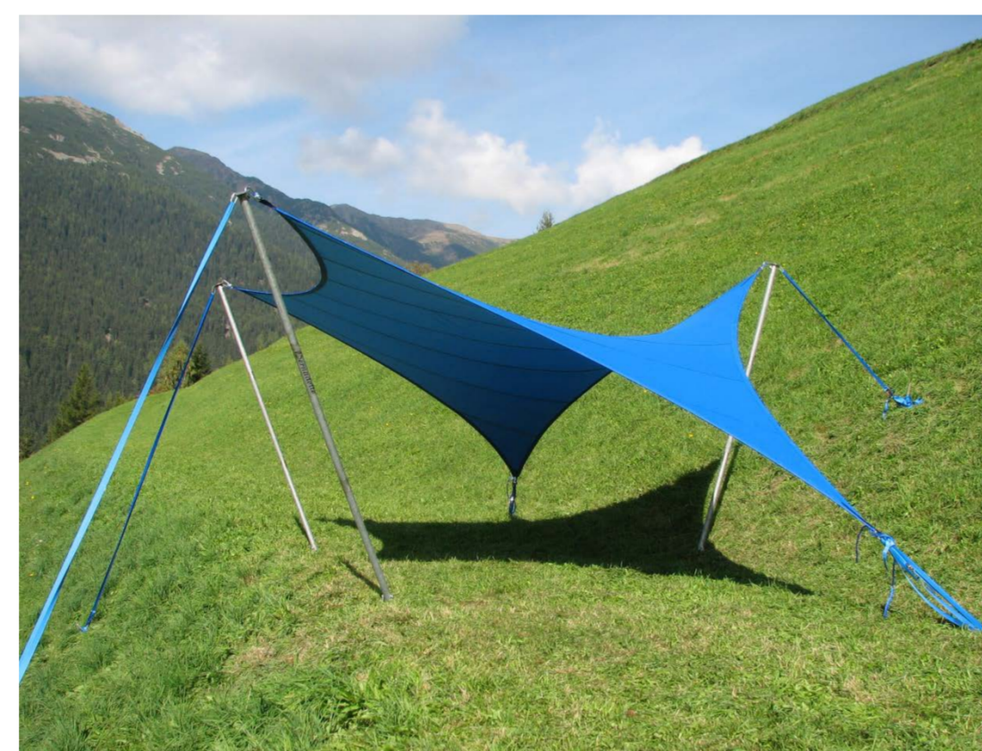
Realization of a 5 point membrane in a student workshop. Form finding and cutting pattern generation
