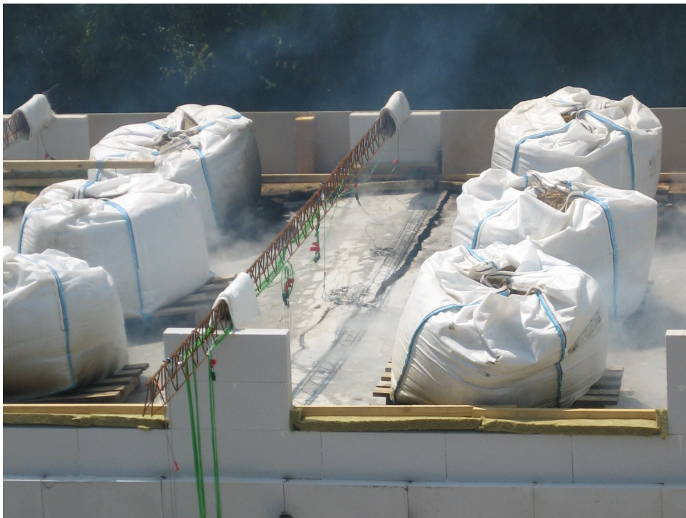
Fig. 2.1: Gaping crack nearby the intermediate beam in first Munich test
