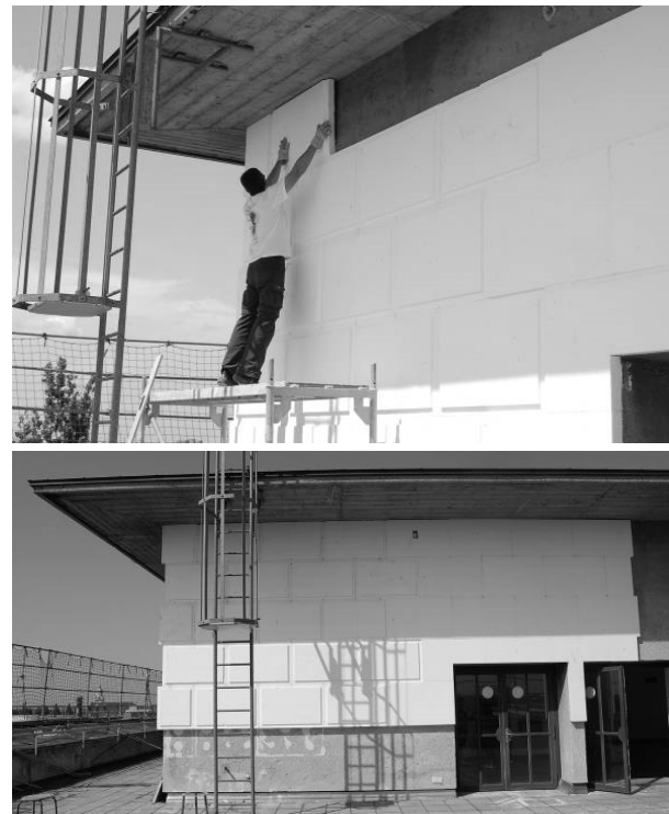
Figure 10: Sample area during mounting work and after completion
