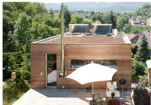
Figure 1: Residential building with wooden flat roof construction
