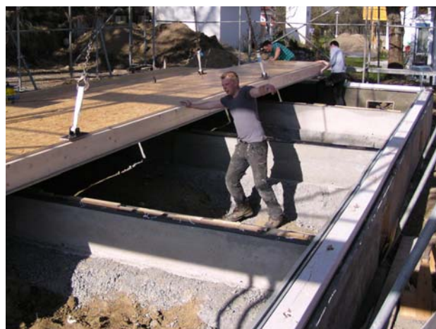
Figure 2: Erection of wooden floor plate on concrete line-foundation
