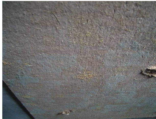
Figure 5: Start of mould on wooden fibre board (07/2007)
