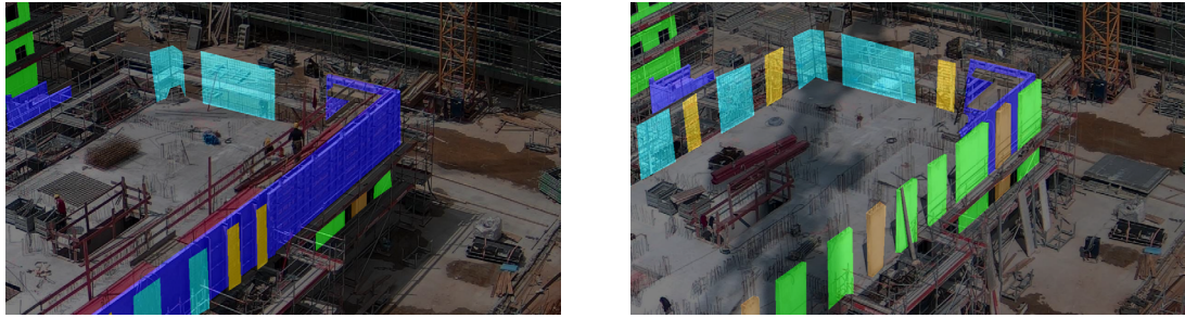
Figure 5.7: Annotation of elements, that are cast together in one formwork during their panel phase (on the left) and their concrete phase (on the right)
