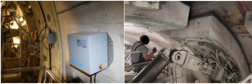
FIGURE 8 Installation of measurement rings U5.
