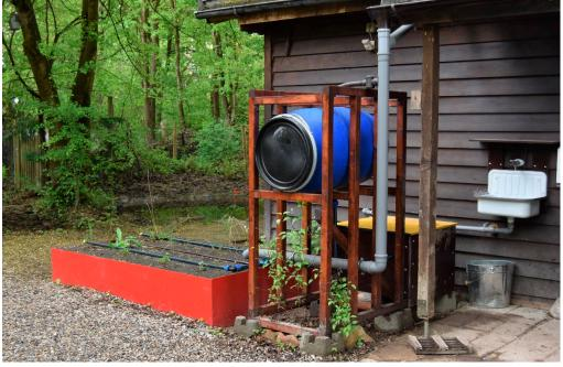
**Figure 14.** Built result of the BGA project 10 months after completion. The operation ran without any disruptions. In winter, the septic tank was bypassed. In the meantime, summer operation was resumed. The plants on the constructed wetland all survived the winter well and will grow even bigger in the next few years.
