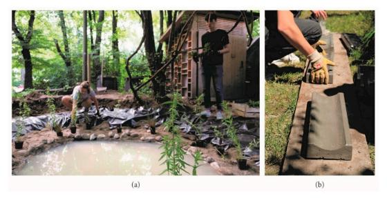
**Figure 12.** (a) The shore zone of the pond is planted with marsh plants. (b) The swale stones are poured and dried on site.
