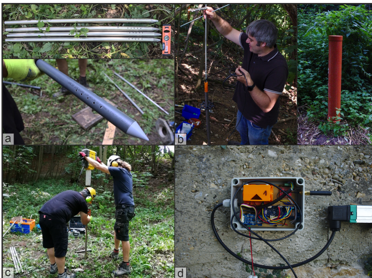
Figure 6. Pictures from a field installation where the presented sensors were tested and evaluated and the installation procedures were developed. (a) Steel and PVC housings with drilled holes for the filter section. (b) Left: installation of sensors into the housing, right: preliminary sensor encasing. (c) Installation of the housing with a jackhammer. (d) Preliminary circuit board for the IN on a wall with attached potentiometer.
