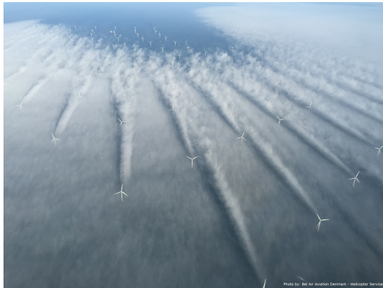
(a) Horns Rev II wind farm off the coast of Denmark. The wake effects are visible due to low hanging fog. Photo by: Bel Air Aviation A/S [12]. January 26th, 2016. Used with permission.
