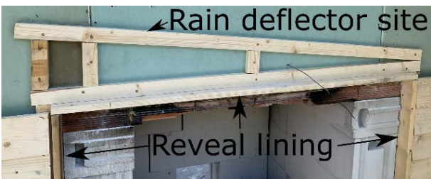
Figure PII. 28 Reveal lining and rain deflector site
