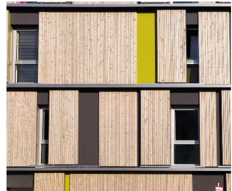
Figure PII. 24 Façade as vertical tongue and groove cladding
