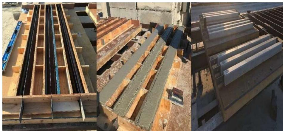
**Figure 5.** The casting of BRB infill with TDA concrete and conventional concrete.
