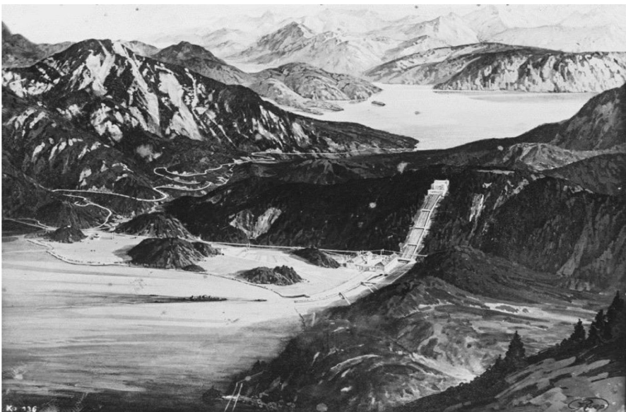
Fig. 1 The Walchensee plant in Upper Bavaria, one of the most iconic major construction projects of the Bavarian energy landscape. The idea to utilize the lake as a high-pressure power reservoir first emerged in the summer of 1904 and was realized in 1924 under the supervision of Oskar von Miller, a Bavarian hydro-engineer (Deutsches Museum Archive)
