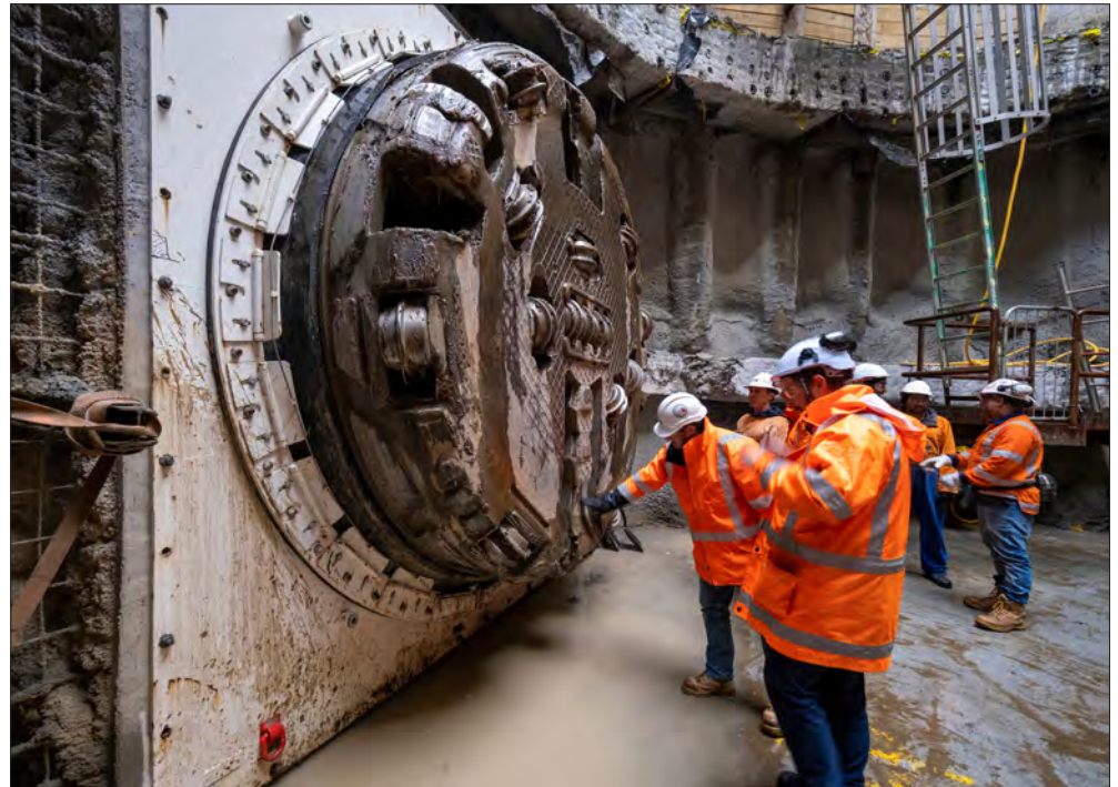
Figure 3. Breakthrough at Hūnua 4 watermain project – drive 2 of 1,296m length. (©McConnell Dowell Constructors Ltd)
