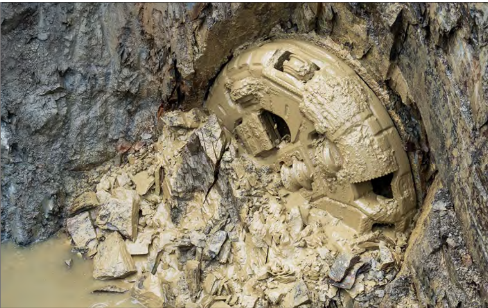
Figure 6. The AVN 1800 before launching the sea outfall drive. (© Eurohinca)
