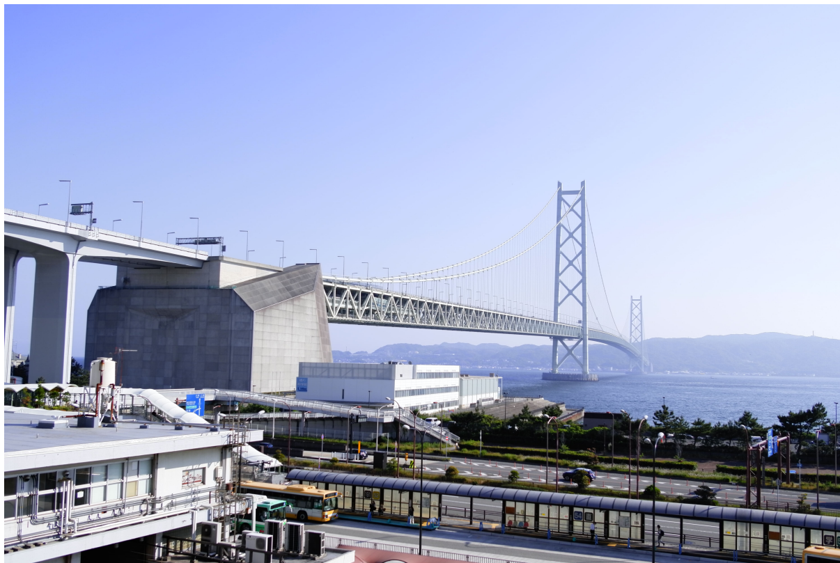
Figure 4: Pioneering application of PCE in concrete: The construction of the Akashi-Kaikyo Bridge (1988-1998) (Photo by Dr. Tsuyoshi Hirata).
