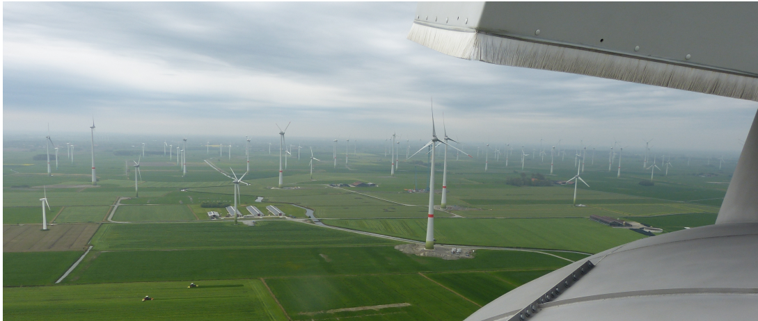
Figure 1: Photograph of Windpark Dornum, taken from PD210 looking towards the south.
