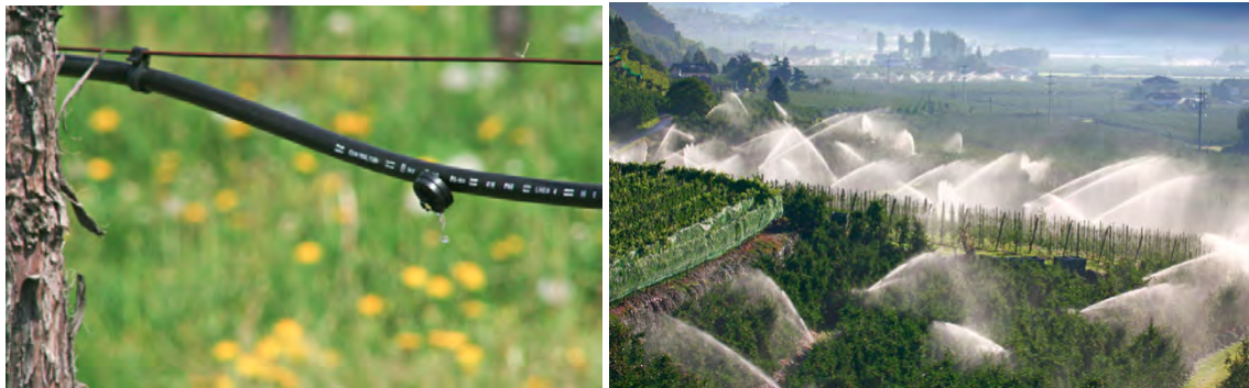
Figure 4.2: Drip and Overhead Irrigation Systems (adopted from Zebisch et al., 2018, p.70)
